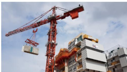
Tower Crane Hoisting of PPVC module
