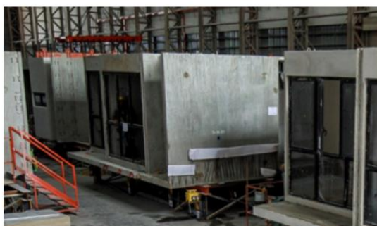
Fit-out Yard Operations
